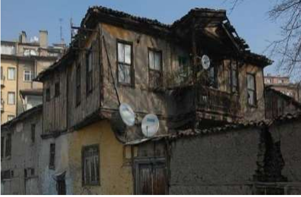
Picture 7. Beynamlızade's Mansion, before restoration (Source: altındag.bel.tr, 2014).
