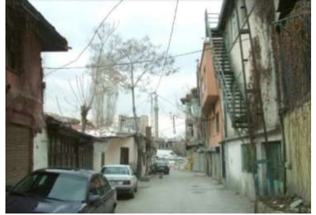
Picture 9. Hamamönü Street, before restoration (Source: altındag.bel.tr, 2014).
