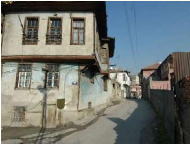
Picture 1. İnci Street, before restoration (Source: altindag.bel.tr,2014)
